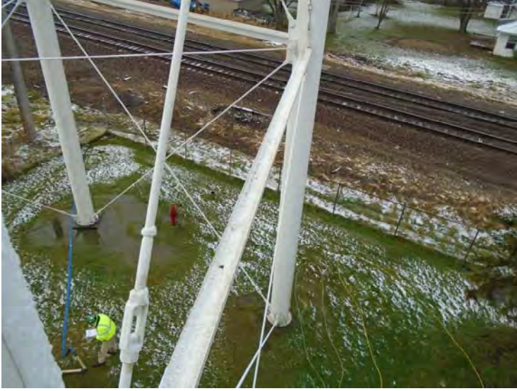
14. The exterior strut coating is in fair condition.
