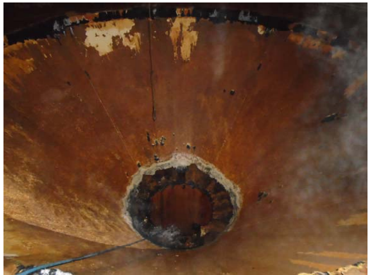
36. Multiple coating breaks were found in the upper transition cone.
