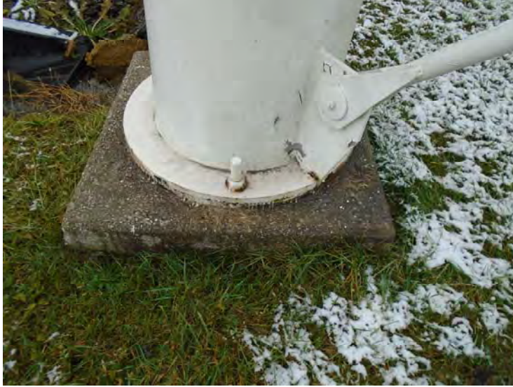
2. The exterior leg foundation is in good condition with minor deterioration.
