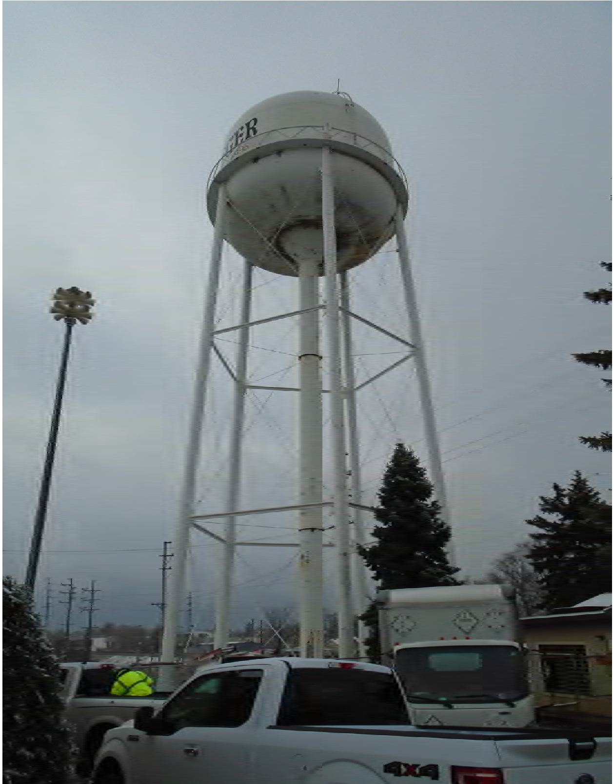
1. The 250,000 gallon torroellipse is located on 31st Street in Steger, Illinois.
