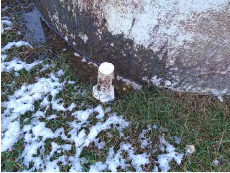
11. The exterior riser anchor bolt coating is in fair condition.
