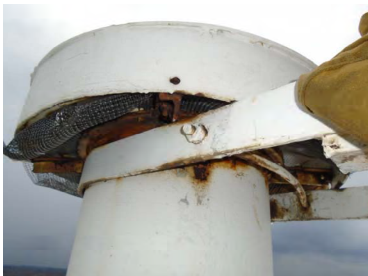
25. The vent screen is in fair condition.
