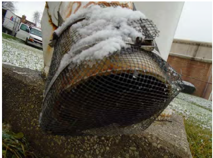
6. The exterior overflow pipe screen is in good condition.
