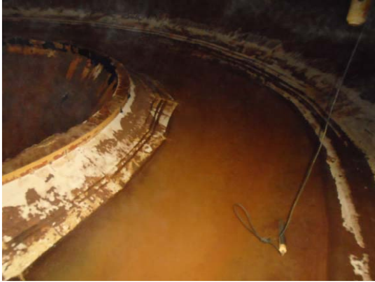
32. Sediment and water was left in the torus prior to the inspection.
