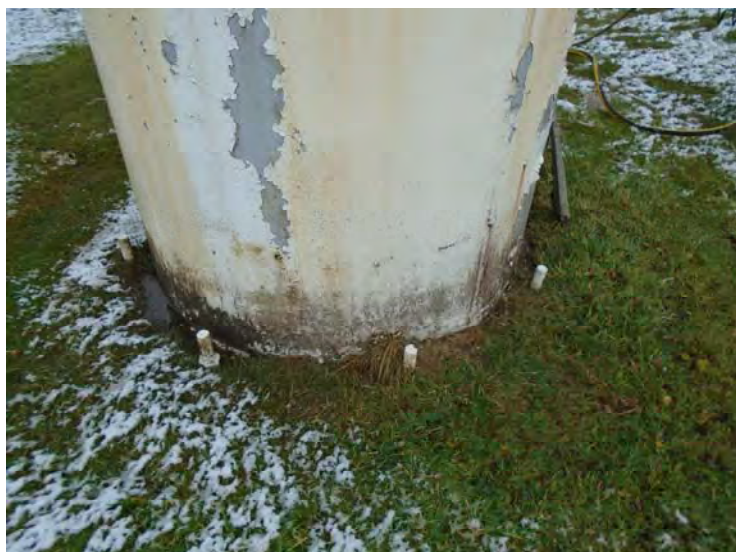
10. The exterior riser foundation is 100% covered with grass and soil.
