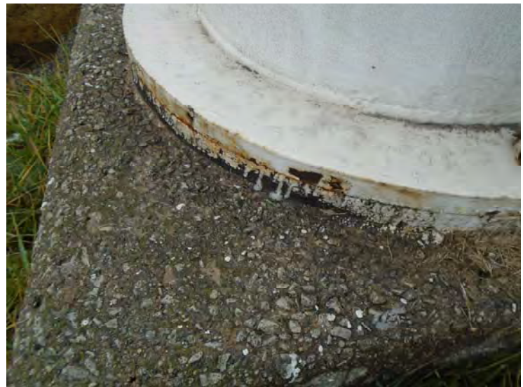
3. The exterior leg grout is in good condition.
