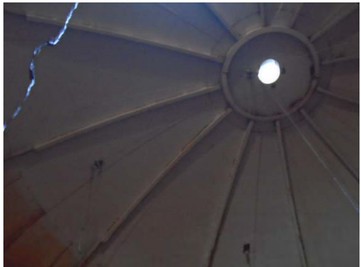
27. The wet interior roof coating is in fair condition.
